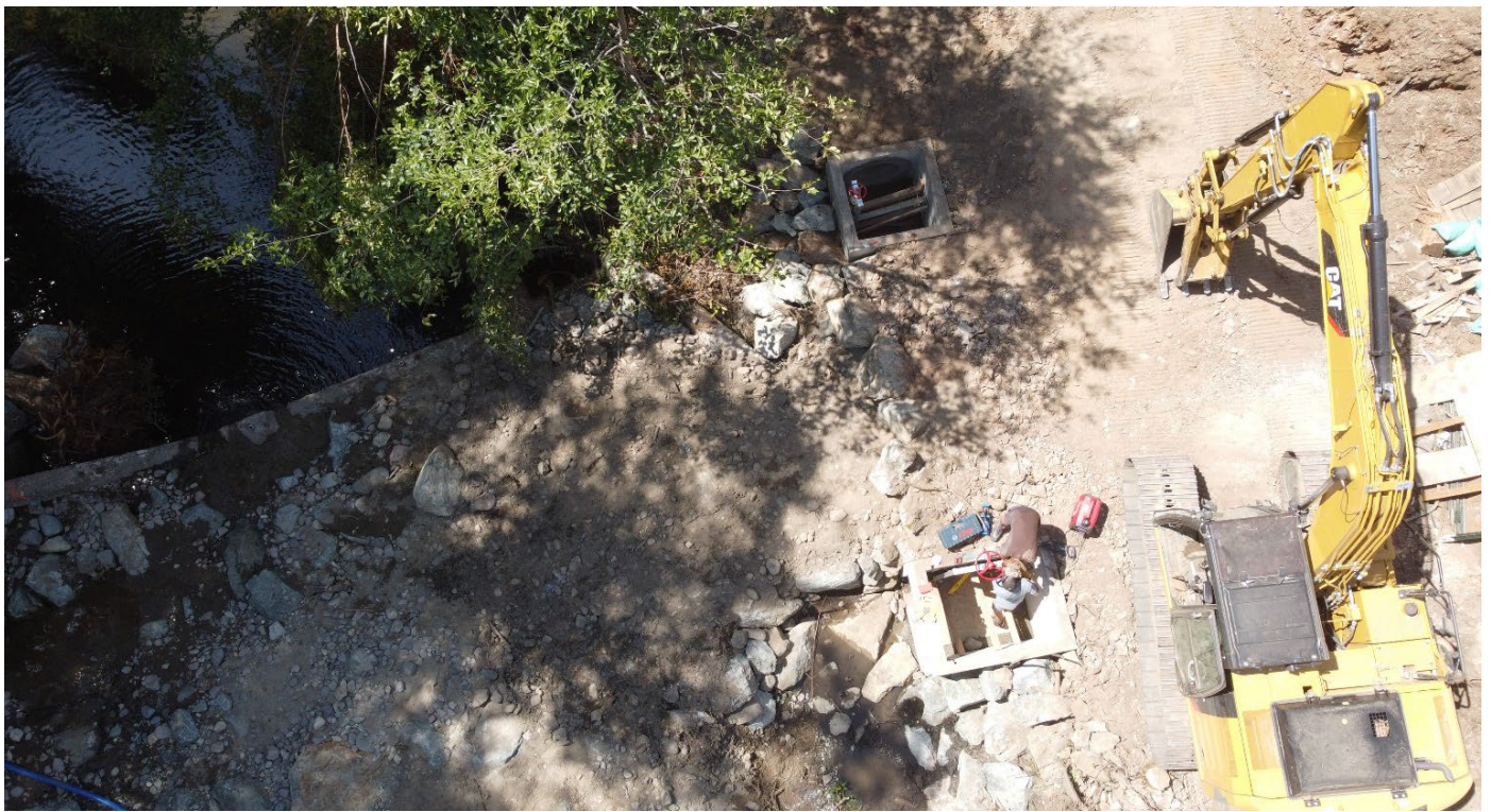
Figure 2. The top photo shows a birdseye view at new headgate during installation at diversion intake on river right. The photo to the right shows construction in progress of log and boulder fish passage and habitat enhancements in river left side channel.
