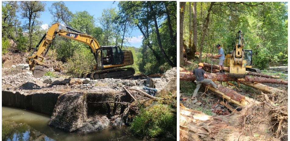
Figure 2. The top photo shows a birdseye view at new headgate during installation at diversion intake on river right. The photo to the right shows construction in progress of log and boulder fish passage and habitat enhancements in river left side channel.
