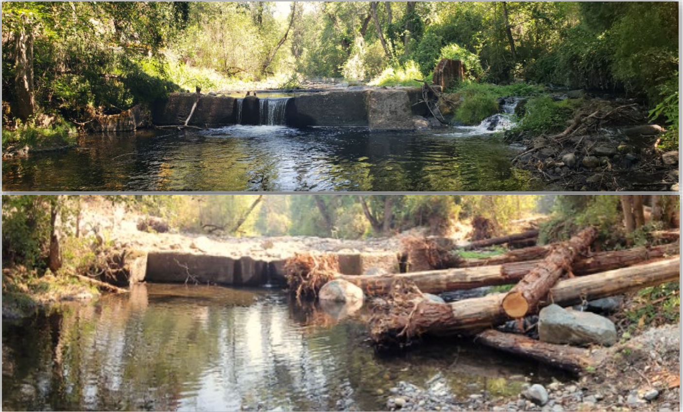
Figure 1. Looking upstream at Upper Phillips Irrigation Diversion on Little Applegate River pre-project in 2021 (top). The second from top shows Upper Phillips after completion of log and boulder fish passage structure and new irrigation headgate (constructed upstream of the concrete dam which remains in place). The lower photos show project components: boulders, concrete pipe, and headgate (left to right).
