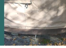
For a secure and comfortable installation, a well-built platform is necessary. To ensure a weather proof installation, the platform needs to be circular and the same diameter as the yurt so the side cover fabric can extend below the interior floor level. This will provide a draft-free and watertight seal. Any exterior decking should be separated from, or at a lower level than the yurt platform.
